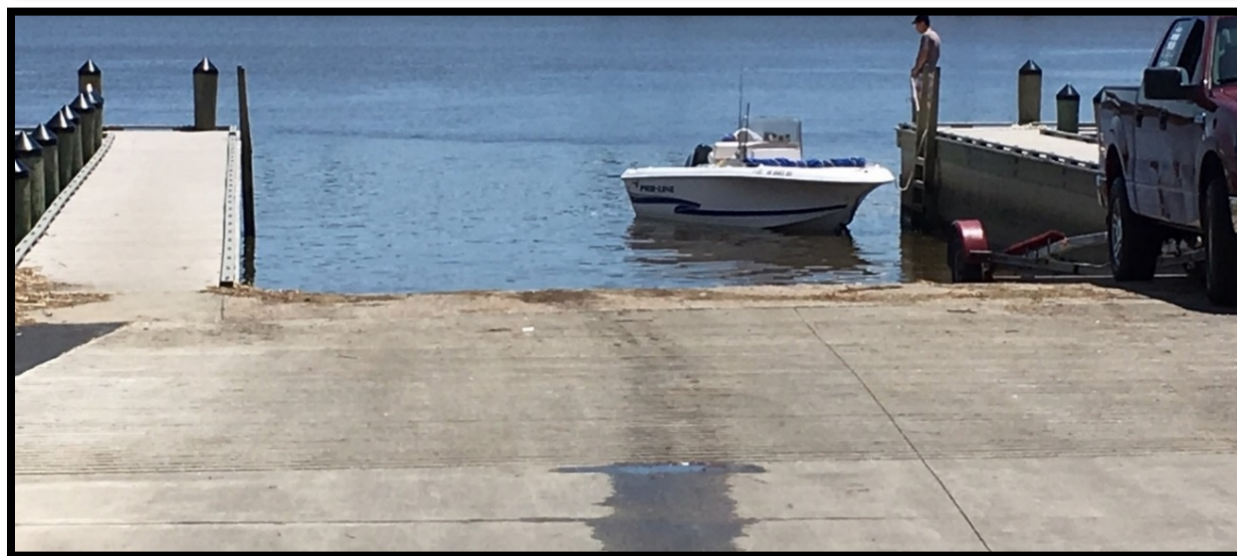
Figures 9a and 9b. West Point BA access facility provides a hardened hand-carry boat ramp (9a) and multiple hardened trailered boat ramps (9b) (West Point River, Virginia). (Credit: John Kirk)
