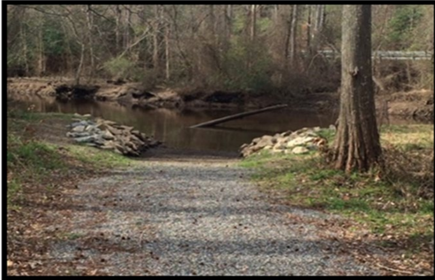
Figure 6. A narrow, pervious surface (e.g., gravel, dirt) water access site designed primarily for hand-carry boats (Morris Creek, Virginia). (Credit: John Kirk)
