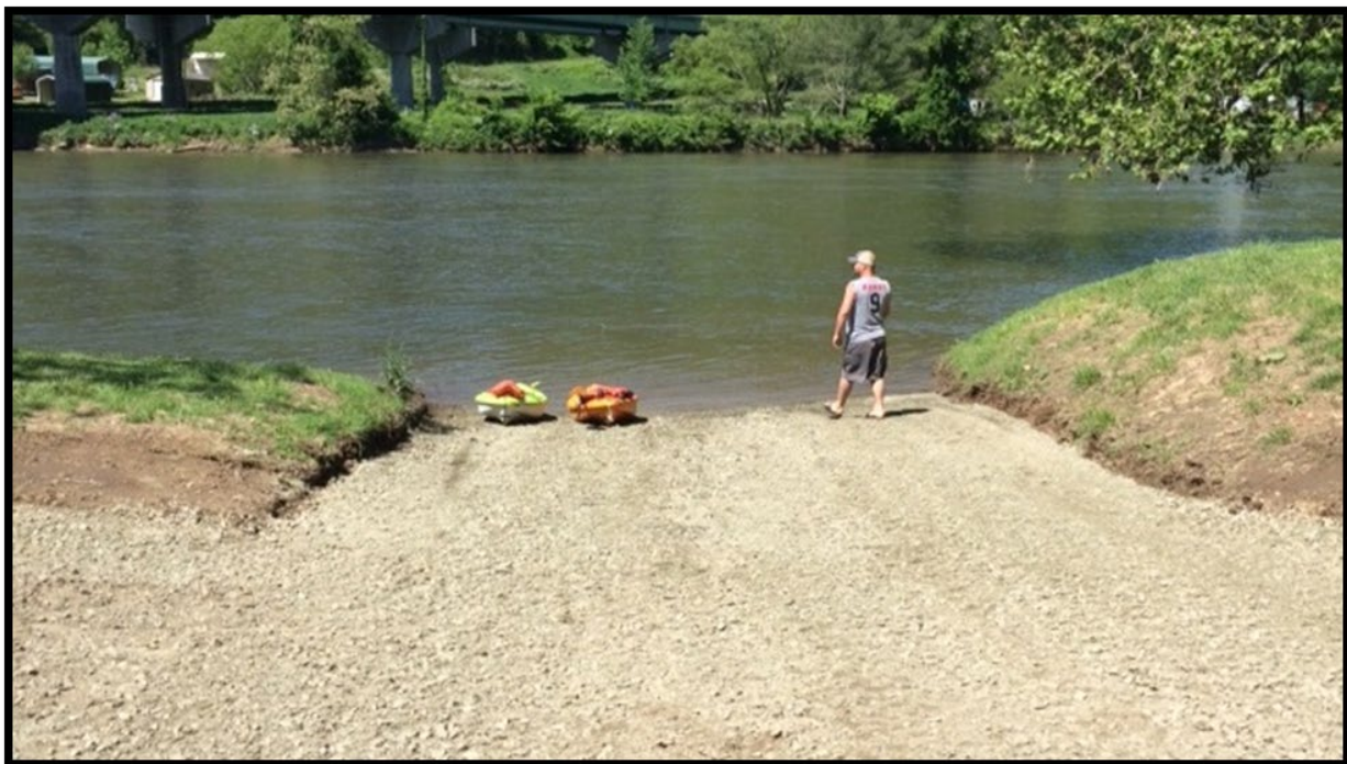
Figure 7. A wider boat launch constructed of pervious surface (e.g., gravel, dirt) with a short concrete slab at the water's edge. This example is primarily designed for hand-carry boats; however, if water levels are appropriate, small, motorized trailered boats also could use this ramp (Baywood on New River, Virginia). (Credit: Toby McClanahan)
