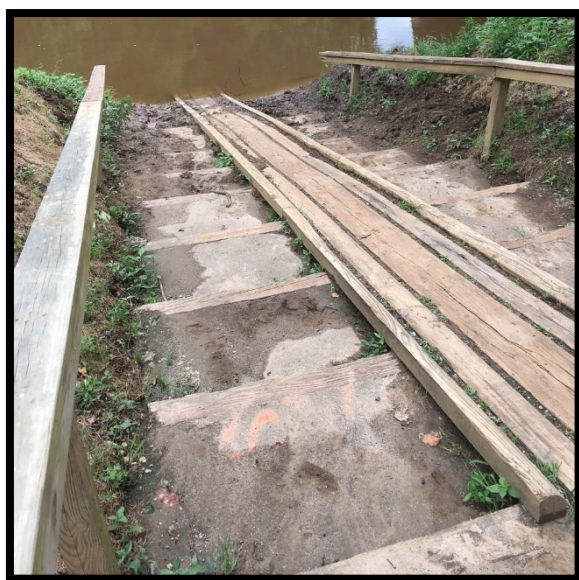
Figure 5. Water access provided via reinforced steps on either side of a wooden boat slide to facilitate launching and retrieving hand-carry boats (Little Page Bridge, Pamunkey River, Virginia). (Credit: John Kirk)
