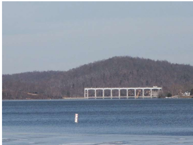
View of Claytor Lake Dam from Claytor Lake State Park's boat ramp.
